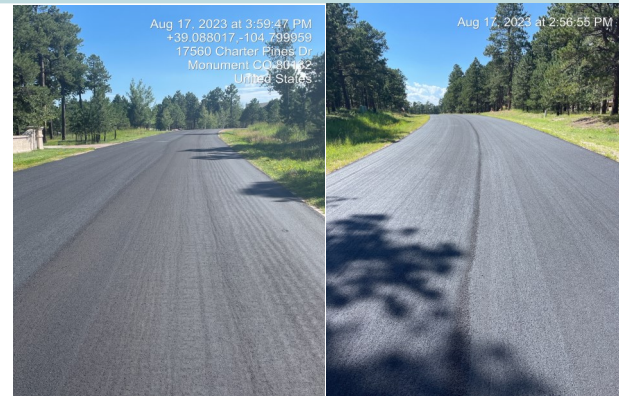
Example of a nearby road that has been slurry sealed.
