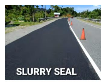
The section of Milam running from Shoup Road to Saxton Hollow Road will be slurry sealed as part of this year's maintenance schedule. (A slurry seal is the application of a mixture of water, asphalt emulsion, very small crushed rock, and additives to an existing asphalt pavement surface.) This section of Milam is not in nearly the same poor condition as the section in Cathedral Pines.
